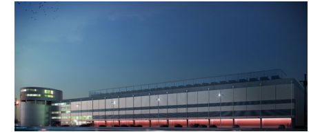
Equinix PA4 IBX exterior
